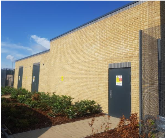
Ipswich Road switch house and transformer enclosure
