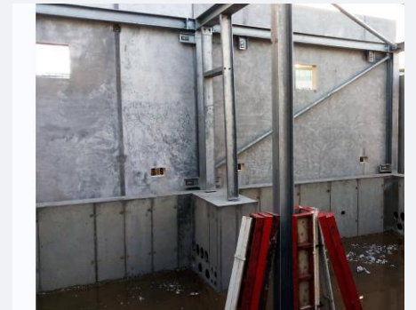
In-Situ Bund, Superstructure and internal PCC Panels
